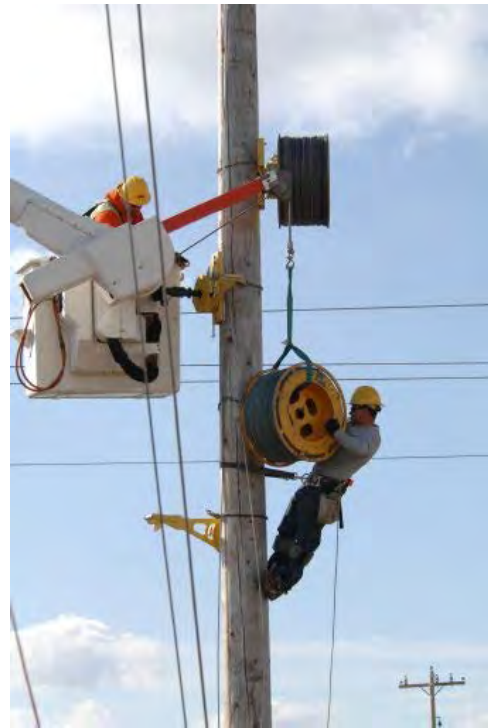
Idaho Power linemen install upgrades.
