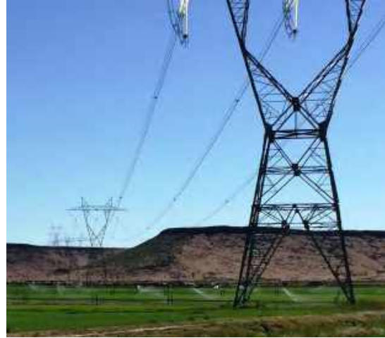
500-kilovolt (kV) transmission line near Melba, Idaho
