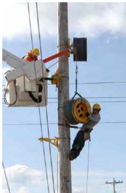
Idaho Power linemen install upgrades.
