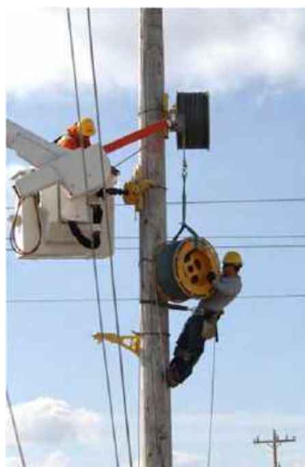
Idaho Power linemen install upgrades.
